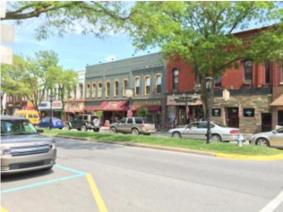
Storefronts in Wellsboro exhibit a consistent scale, retain classic elements and showcase decorative work.
