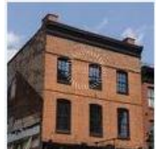
Building with concealed cell tower (Photo Credit: Stealth Concealment)
